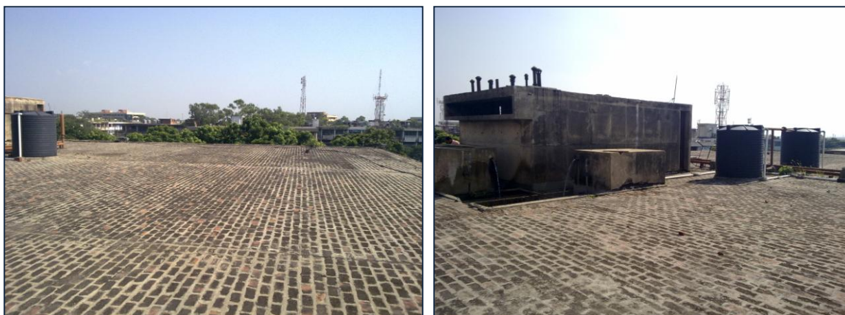
Figure 1: Picture of the roof top of ATH building
